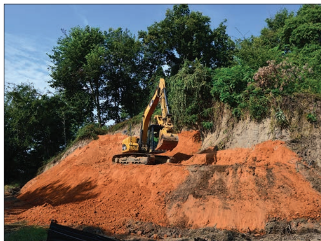
Archeologists monitored as heavy equipment was used first to clean the east side of Cavanaugh Mound in Fort Smith so a profile of mound construction could be observed, then as soil was added to rebuild and stabilize the mound, preventing further erosion (ARAS-UAFS DSC-1751 and DSC_1807, 2017, digital photos by Tim Mulvihill).
